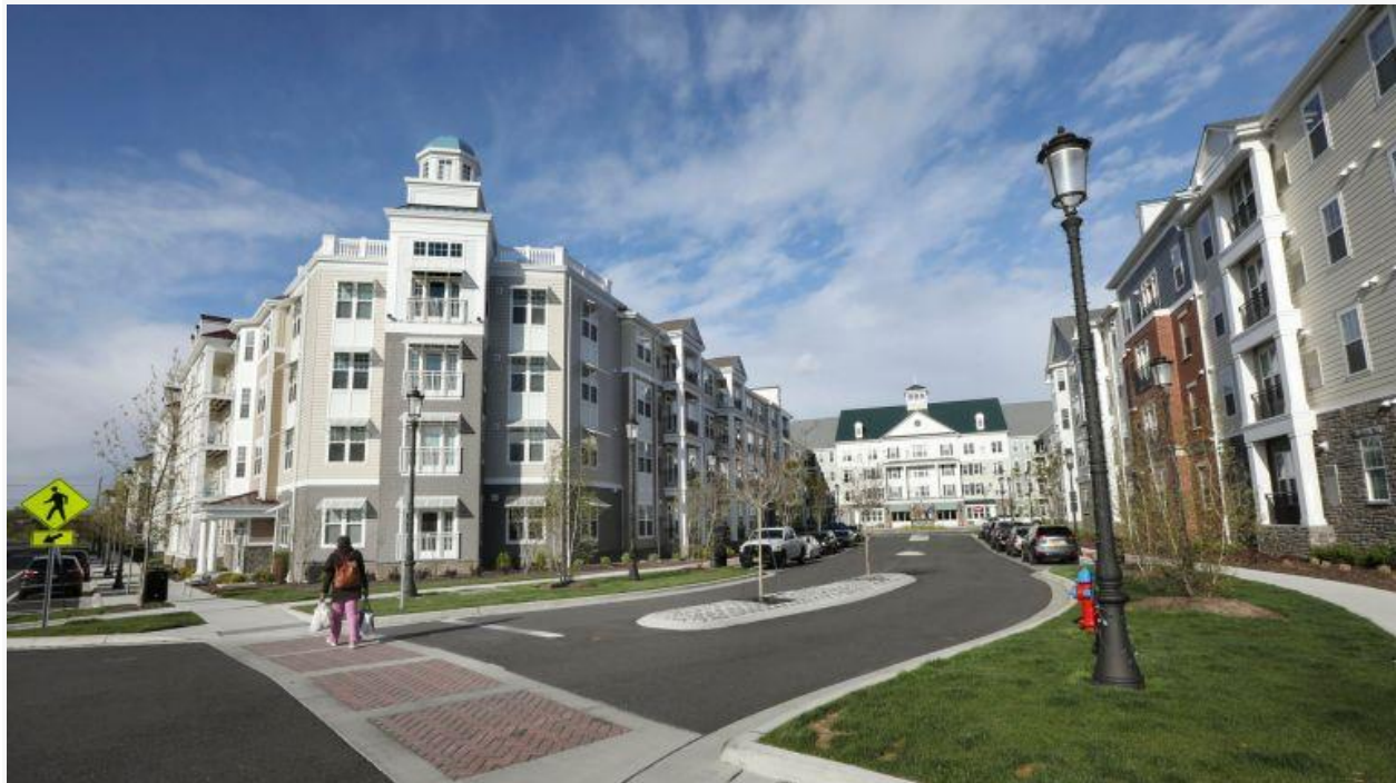
The new Alston Station Square apartments off Mill Road at the Ronkonkoma Hub, are seen on Saturday, May 9, 2020. Credit: Newsday/John Paraskevas
