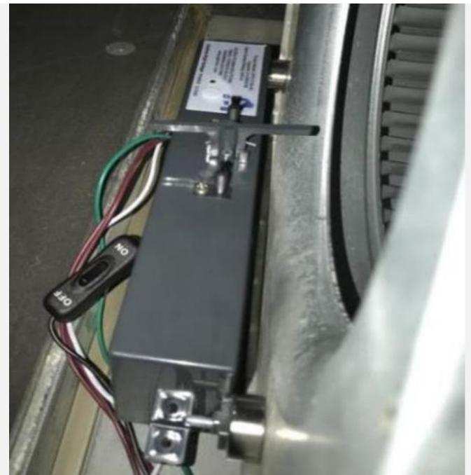
The plan to improve indoor air quality at Mastercard's Headquarters in NYC included the installation of an O<sub>2</sub>Prime Needlepoint Bipolar Ionization. This provided the benefits of no retro-fit costs, less pressure drop, and less energy usage, without generating ozone.
