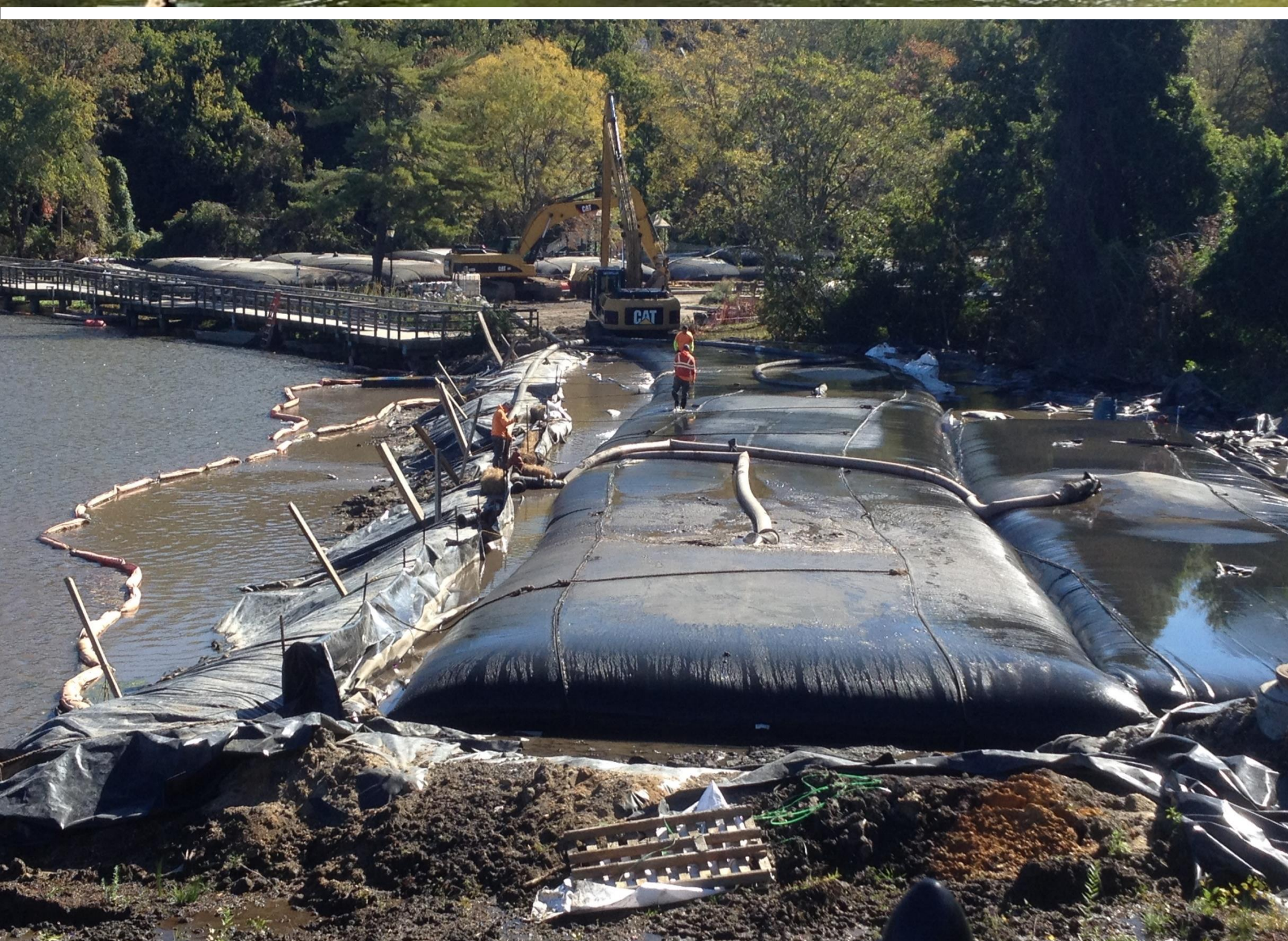
Geotubes containing dredged soils
