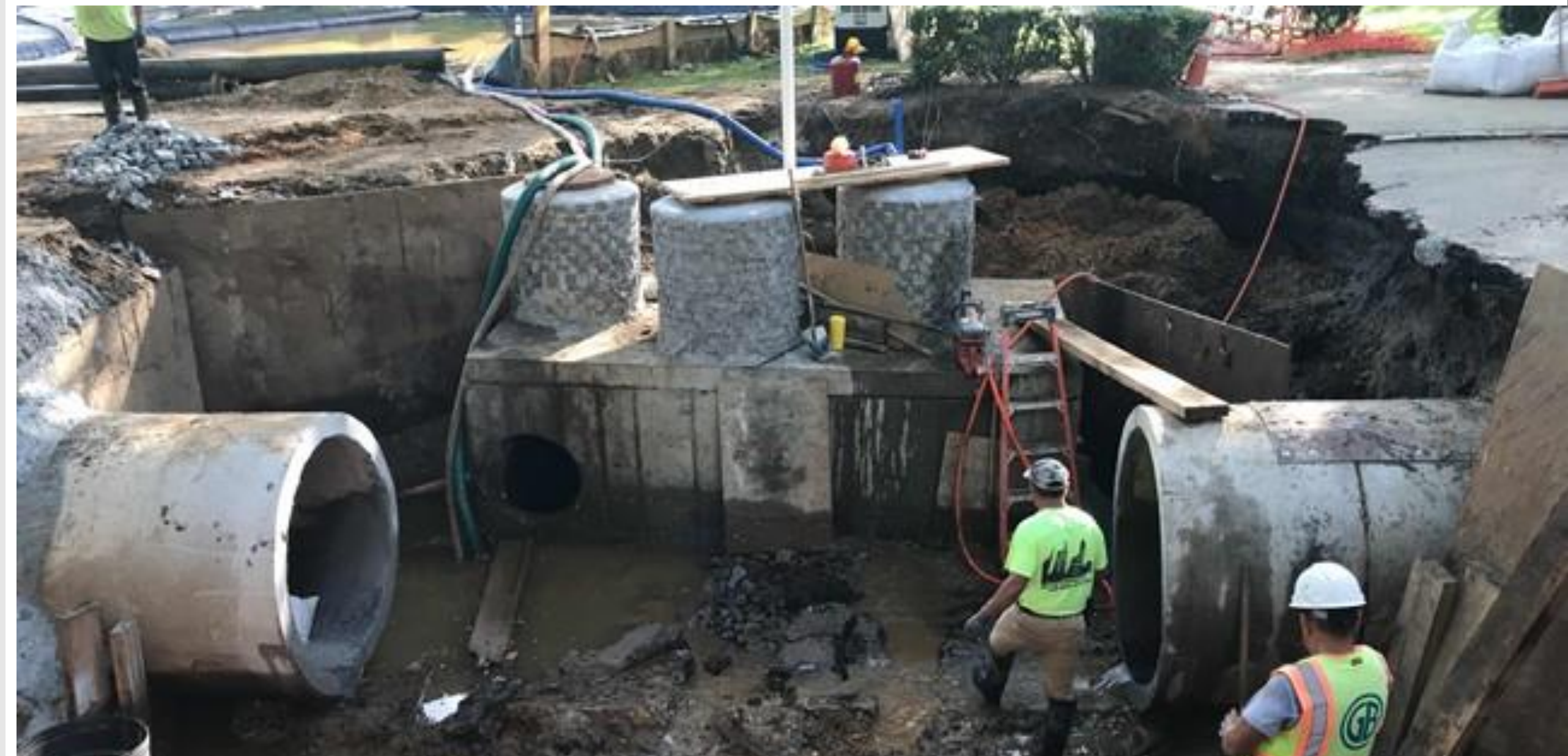
Installation of Stormwater Chamber
