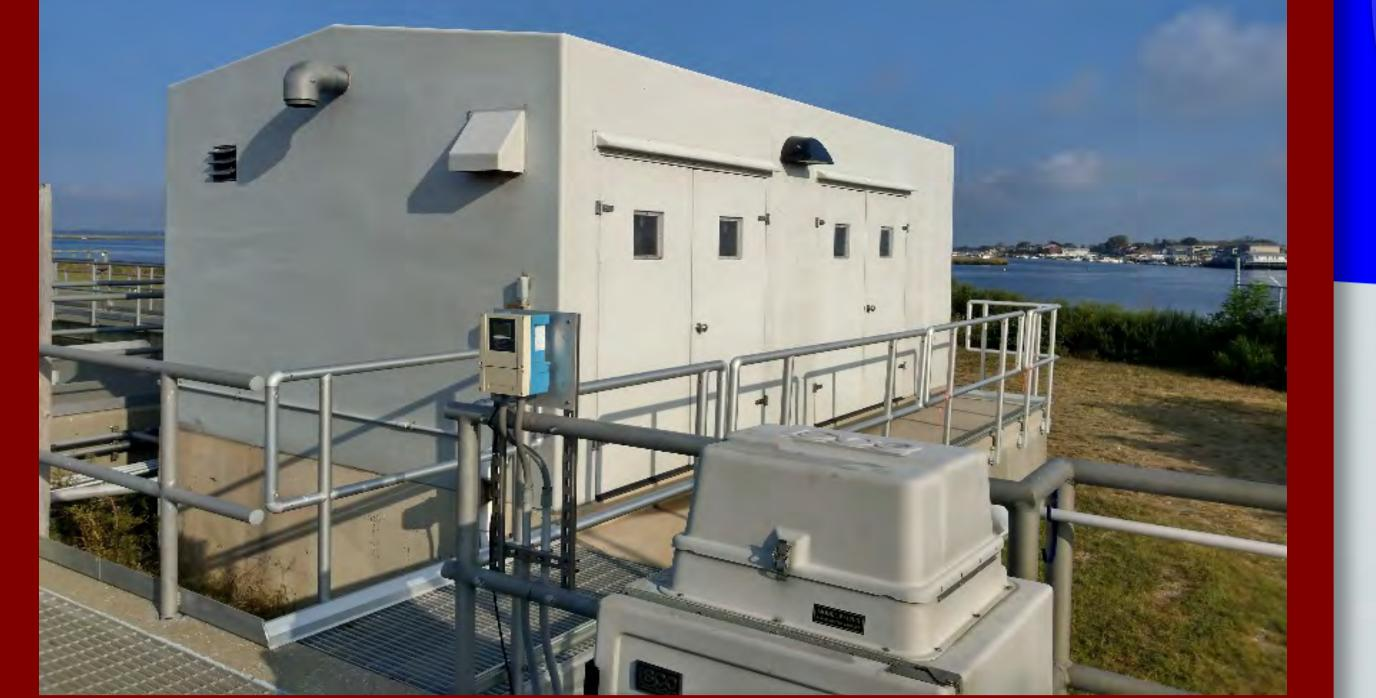
Effluent chlorine probe measures residual chlorine concentrations
