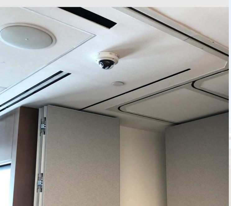
The AV system has partition sensors for the operable walls that can detect when the room is fully open or partitioned off enabling the AV controls to adjust automatically.
