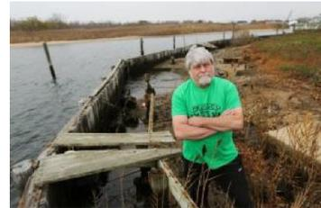
Miles of wooden bulkheads protecting Long Island waterfront properties from erosion are nearing the end of their useful life span — rotting, rusting and below current height codes.
